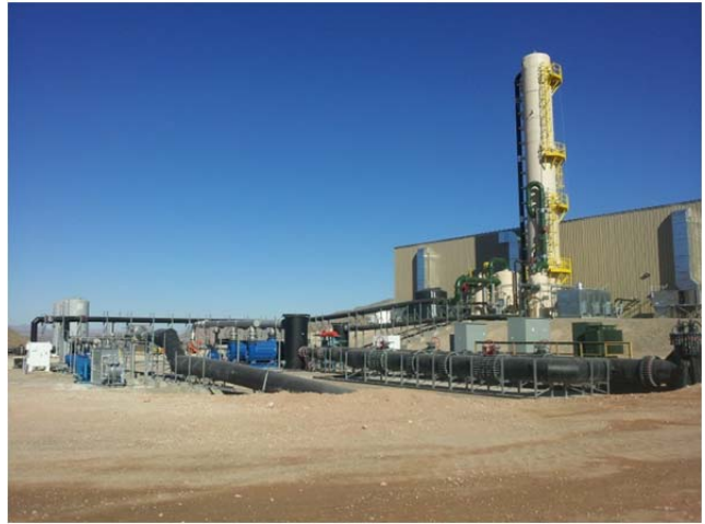
FIGURE 4 VIEW OF THE NEW FLARE STATION AND BIO- DESULFURIZATION PLANT
