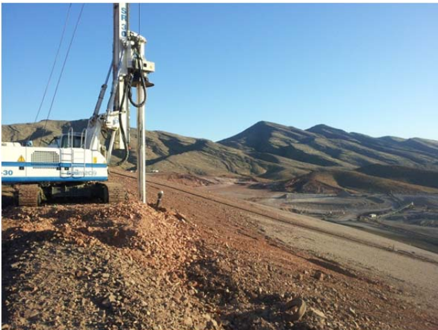
FIGURE 3 VERTICAL GAS EXTRACTION WELL DRILLING
