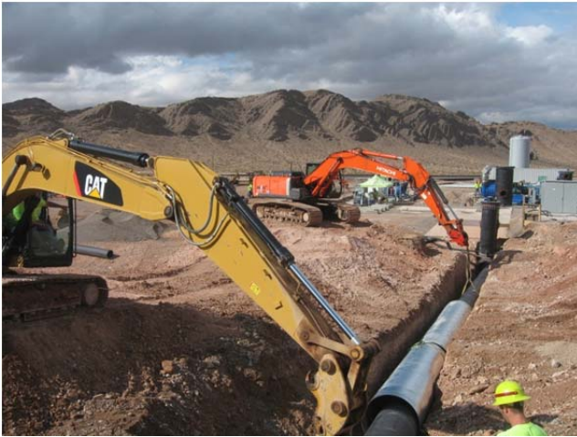
FIGURE 2 INSTALLATION OF NEW 36-INCH FLARE STATION INLET HEADER
