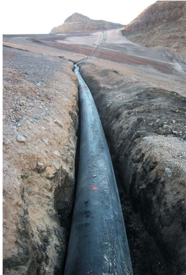
FIGURE 1 INSTALLATION OF 24-INCH WELLFIELD HEADER
